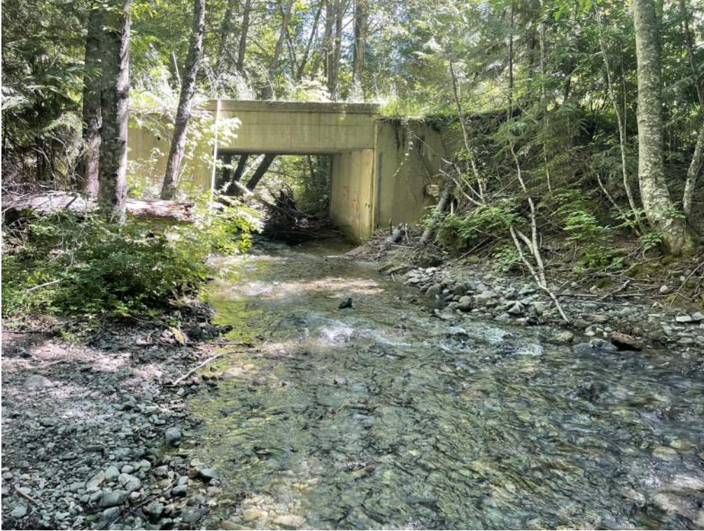
Photograph 7: Little Creek looking downstream. Photo taken July 2022.
