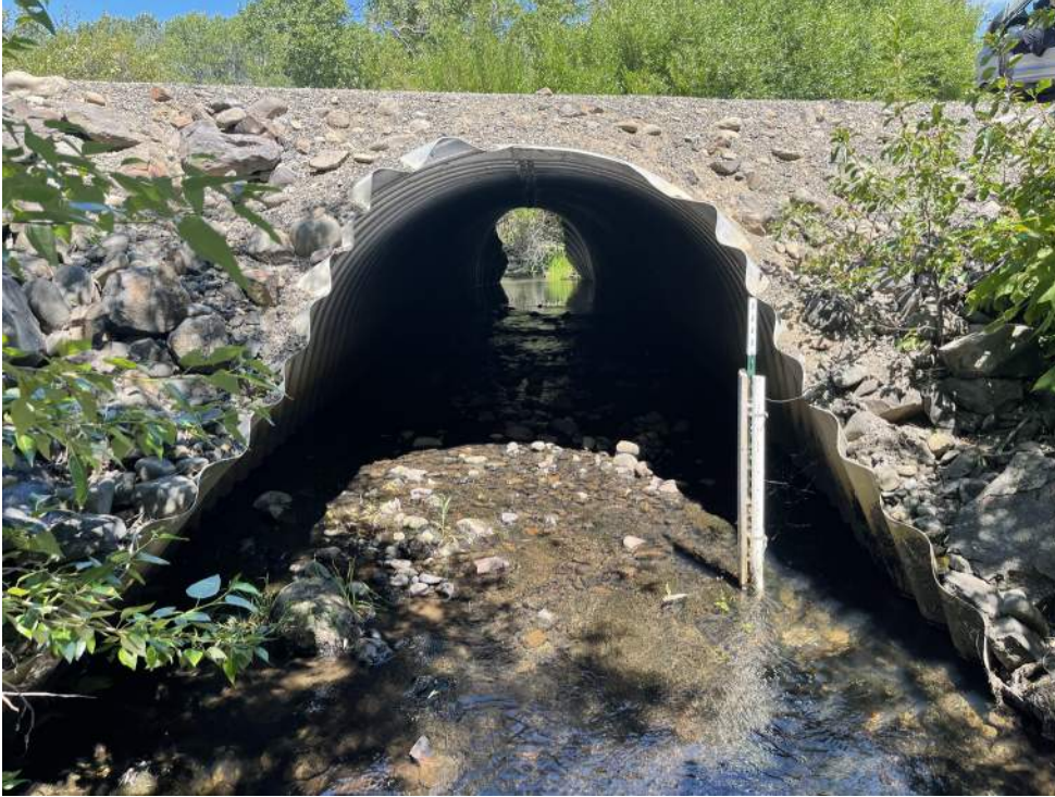
Photograph 13: Wilson Creek looking upstream. Photo taken July 2022.
